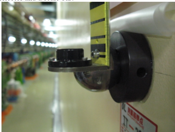
Figure 4: Newly installed wall monument.
