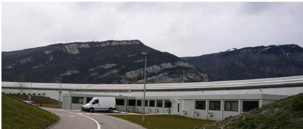
Figure 7 Over a relatively short time in summer 2008 roughly 6000 m 3 (12 kT) of earth was moved from the site where the buildings now stand to the adjacent areas. A net upward movement of 225 \mu\text{m} was registered on an HLS installed on the SR tunnel roof located roughly 60 to 70 m away.
