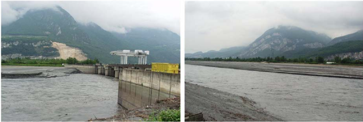
Figure 6 The purging of the St Egrève dam downriver of the ESRF causes permanent site uplift and subsidence movements in the order \pm 150 \mu\text{m} . The top graph shows this movement at one point measured by the HLS installed on the SR tunnel roof. The bottom two photos show the dam and sediment in the Isère River.
