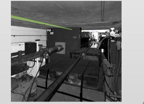
In the undulator hall a battery of sensors (hydrostatic leveling sensors and wire position monitors) is used to monitor the position of 33 girders.
